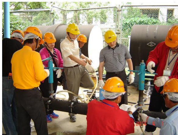
Training course of water piping works
