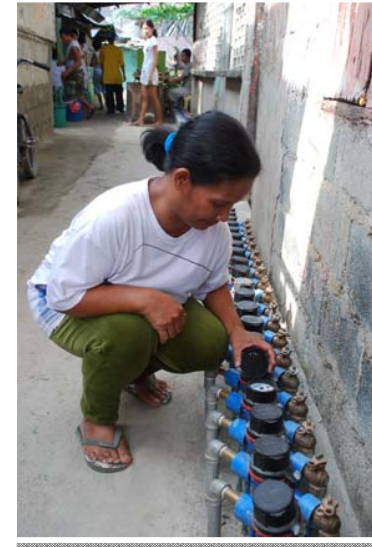
REGULAR WATER SERVICE CONNECTIONS
