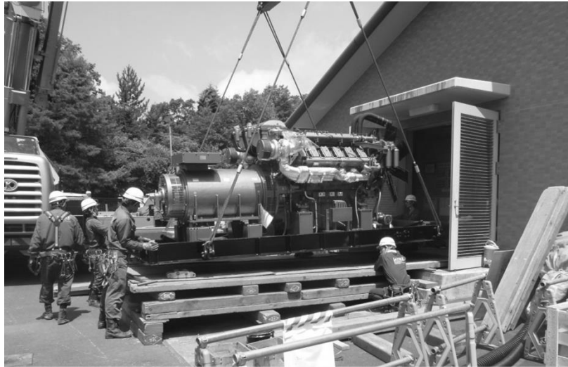
Figure 3. The upgrade construction in Tsunakizaka Water Supply Pump Station
