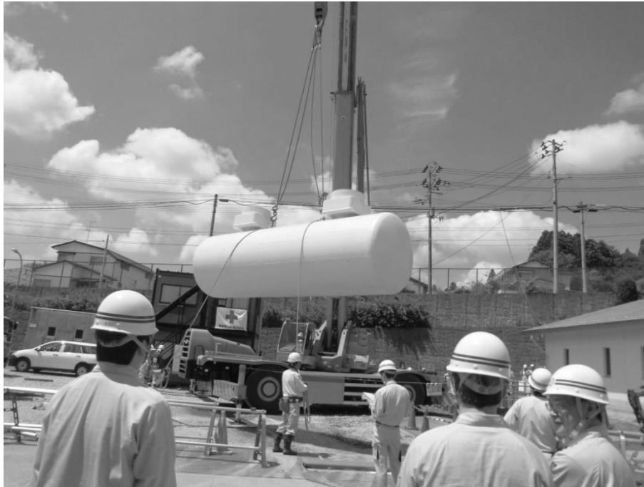
Figure 2. The expansion works in Kunimi Water Purification Plant
